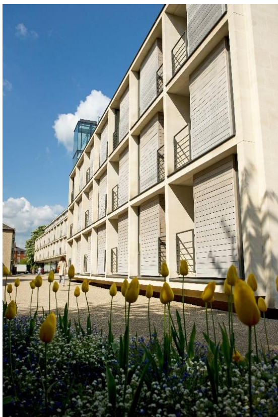
Exterior of the Ruth Deech Building
